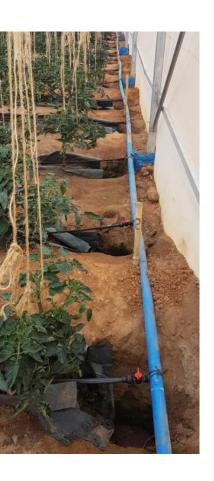
Before they can install the Mtumbwi we check the slope/drain, we have an slope of 3%, means on 20 meter 60 cm different.
