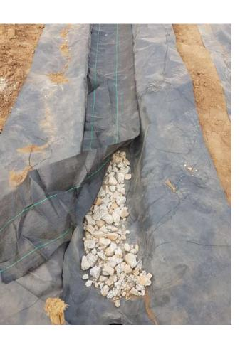
After the slope/drain is inline, we add at the bottem an we add an layer of ground cover quality 160gr/m2, after this the plastic 200 micron.
